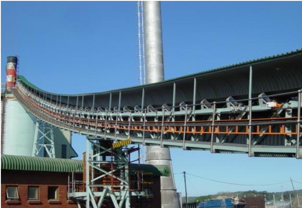
Figure 12: Biomass Feed Conveyor, Tugela Mill Fuel Switching Project
