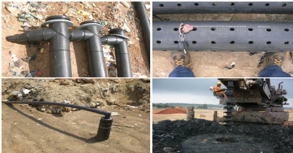
Figure 14: Wells installed at EnviroServ Chloorkop Landfill Site
